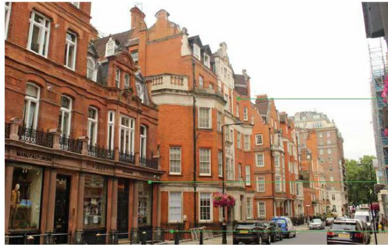
View from the corner to Mount Street and South Audley Street looking towards the
